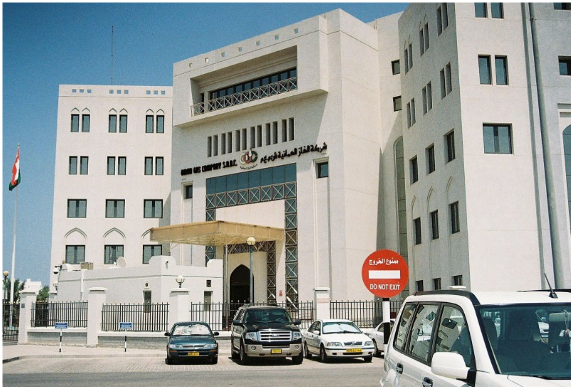
Oman Gas Company (Photo by Flow Research)
