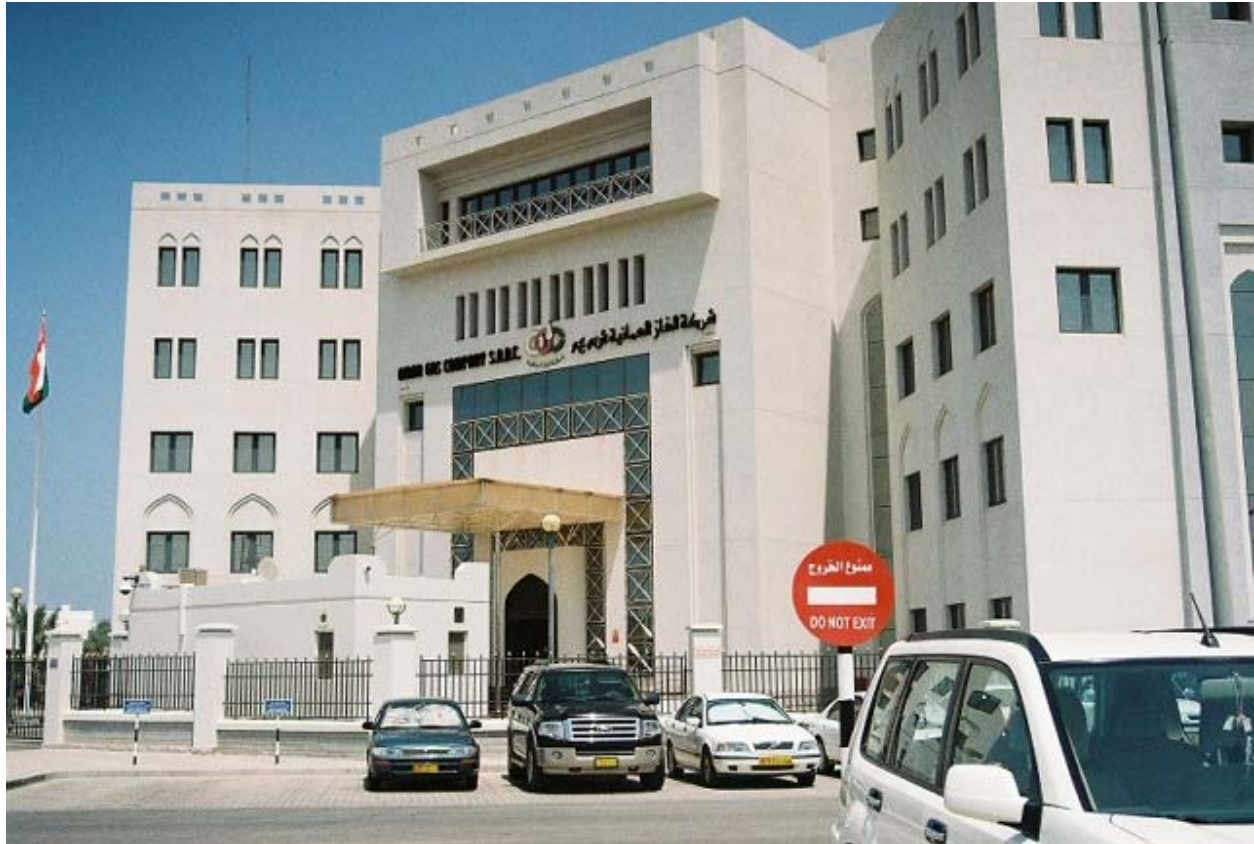
Above: Oman Gas Company Photo by Flow Research
