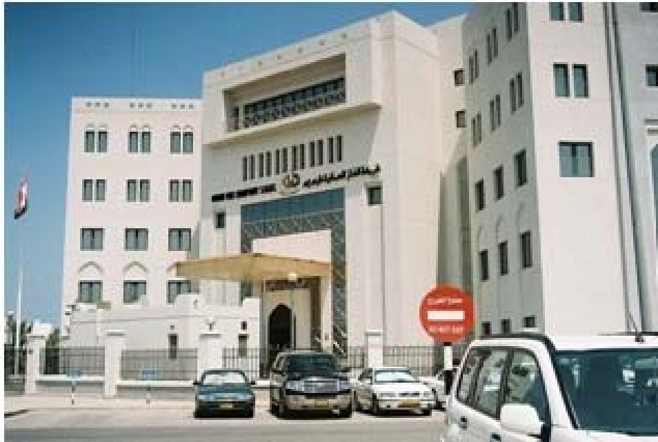
OMAN Gas Company Photo by Flow Research
